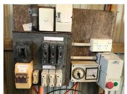
The main pump shed recently had an electrical upgrade with a new inverter and a new switchboard installed. The inverter was faulty and had to be replaced and the switchboard was
